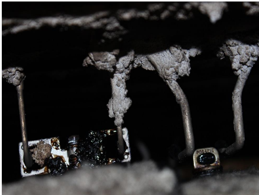
Photo No. 7 Brick Anchors and Ties (After Exposures)
