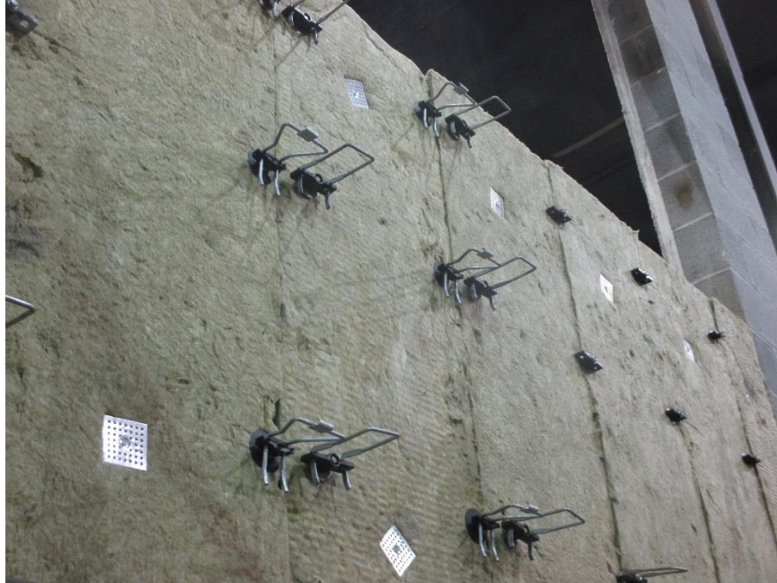
Photo No. 1 Anchor Installation
